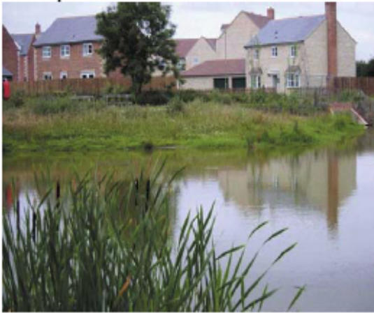
SUDS pond, housing development, Bicester
